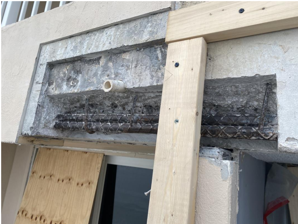
Picture 2: Unit 405 window header repair
