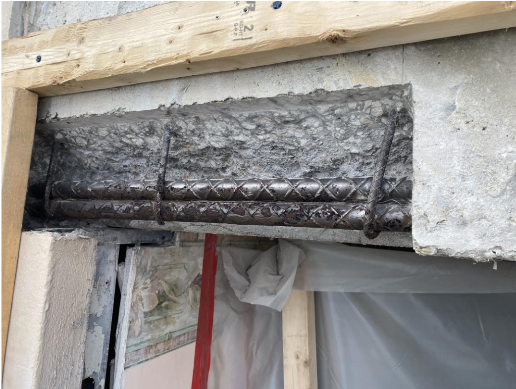
Picture 3: Unit 305 window header repair
