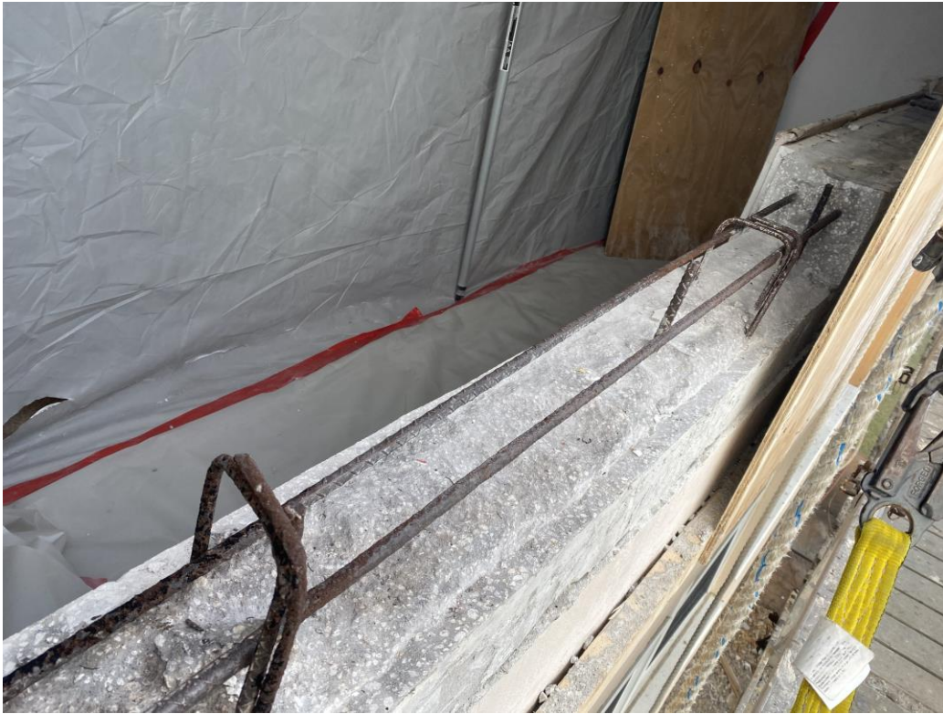
Picture 1: Unit 203 window sill repair
