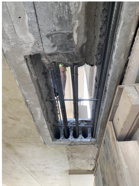
Picture 4: 4 th floor walkway repair
